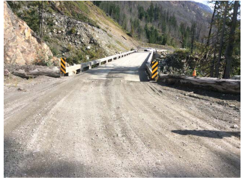
Approach from Right Bank when facing downstream
