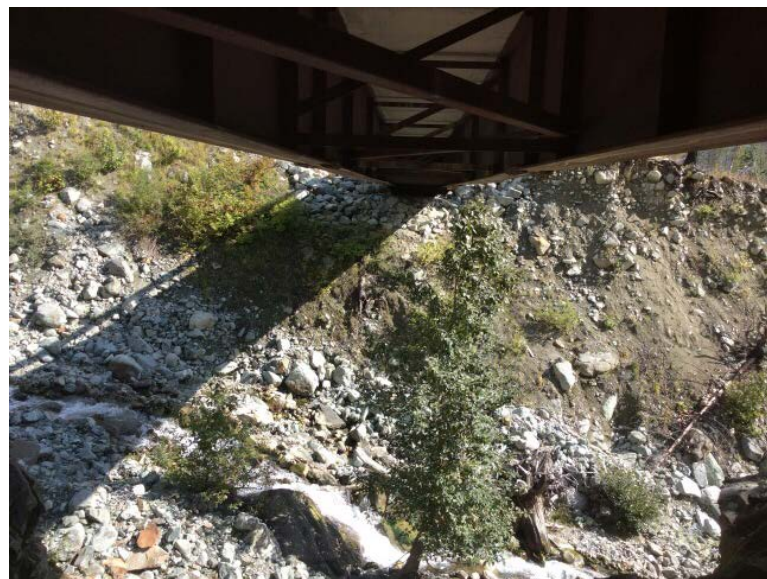
Left Bank Abutment when facing downstream
