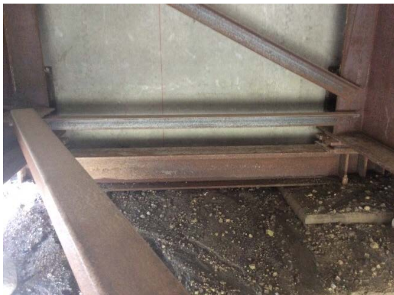
Right Bank Abutment when facing downstream
